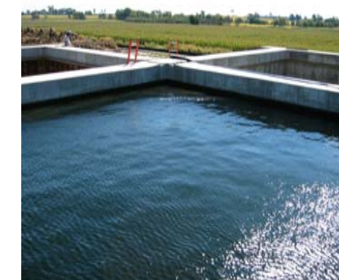
Testing The Tanks
