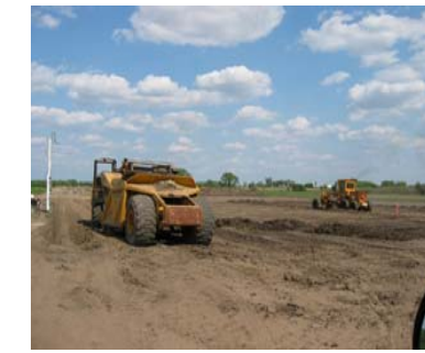
Preparing The Site
