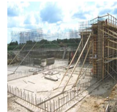
Forming The Walls
